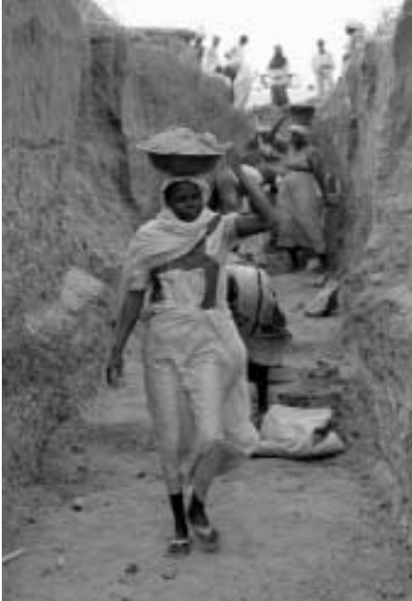
Constructing a traditional hand-dug reservoir ( hafir ) in Sudan
